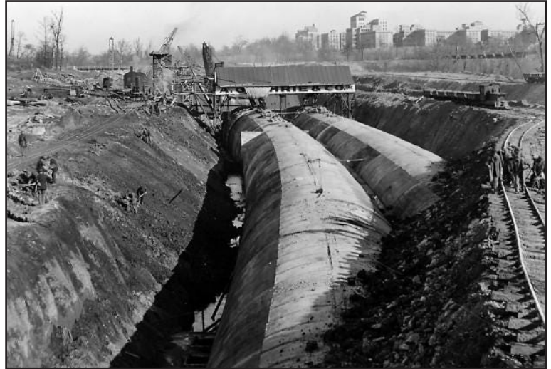
Following the flooding in 1915, portions of the River des Peres running through Forest Park were rerouted through large underground tunnels. Photo from the St. Louis Post-Dispatch.
